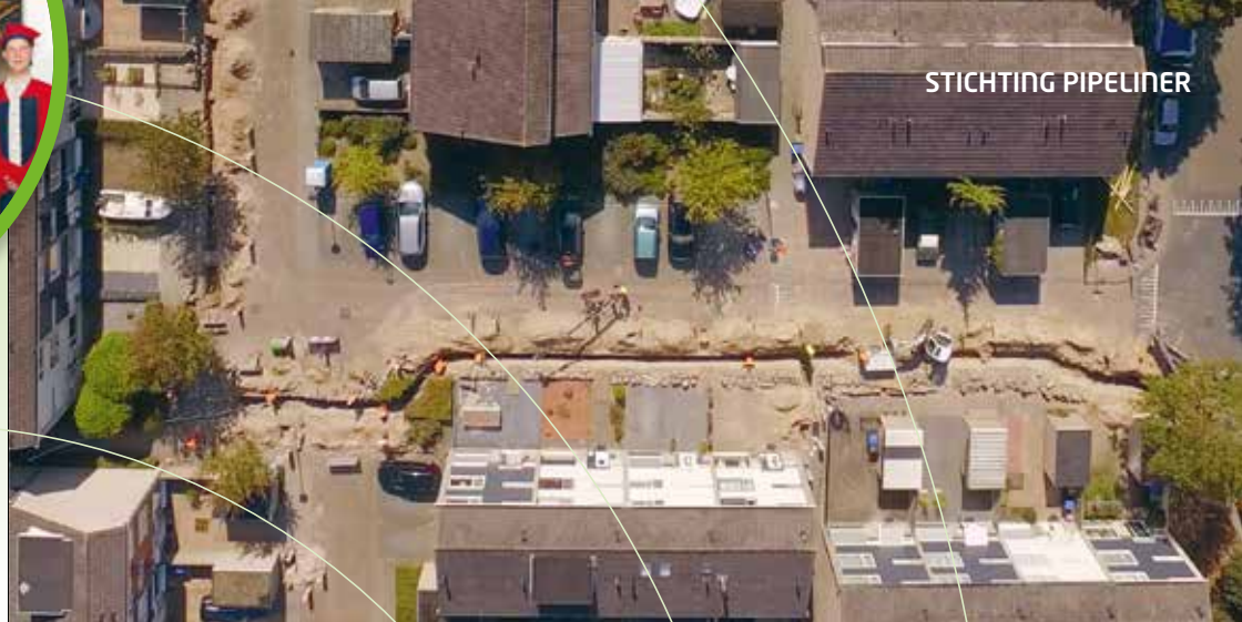
Vernieuwing drinkwaterdistributienet Brabant Water
